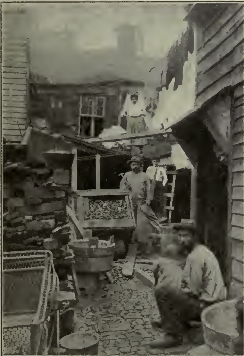
DILAPIDATED HOUSES AND YARD CONDITIONS
